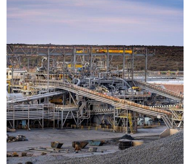
Mount Keith Mine Site (2022)
