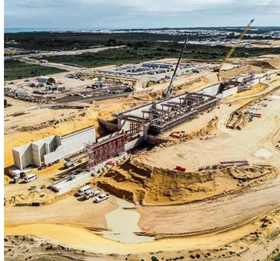
Alkimos Train Station (2023)
